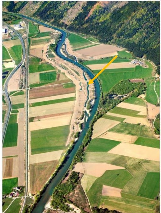
Baufortschritt Flug v. 20.April 2011
